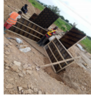
FORM WORK (CULVERT)
