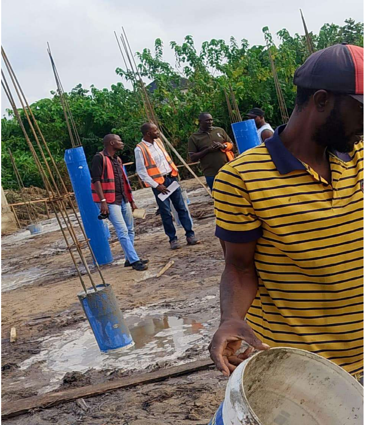
Fig 4.2 Pilling working at Obadore, Lagos during LABSCA visit for stage inspection
