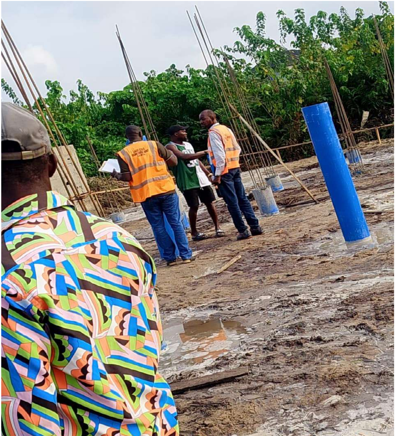
Fig 4.1 Pilling working at Obadore, Lagos during LABSCA visit for stage inspection
