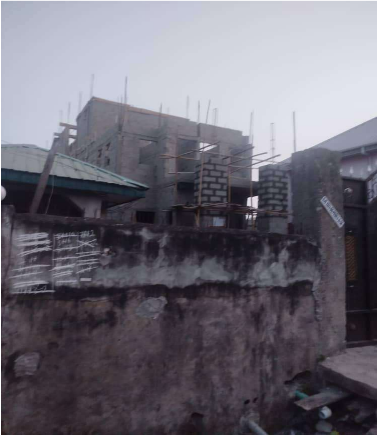
Fig 3.2 Project at Akinjiri Street, Tedi, Lagos
