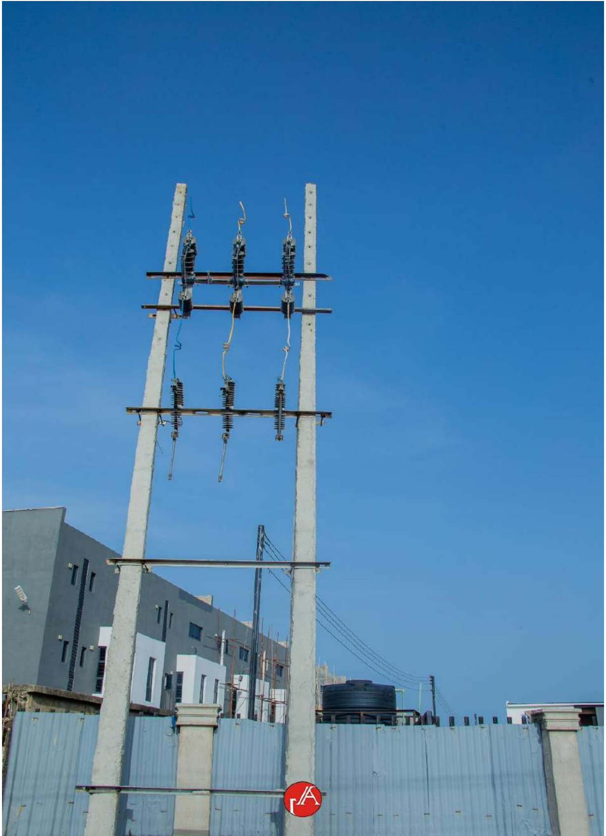
Fig. 13 Installation of HT & LT Line at Orchid 1
