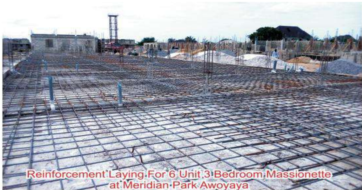
Fig. 2 Reinforcement Laying at Meridian Park Awoyaya for a 6 Unit 3 Bedroom Maisonette
