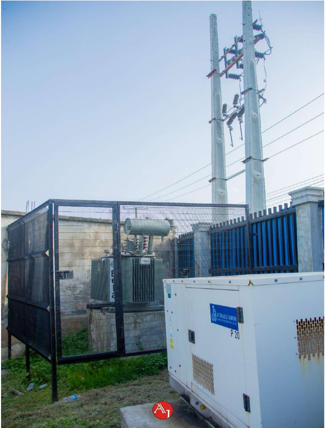
Fig. 12 Installation of 500KVA Transformer at Orchid 1
