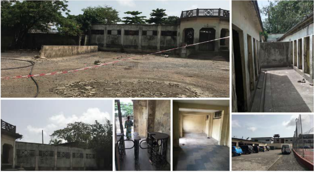
Showing images of the center before redevelopment.
