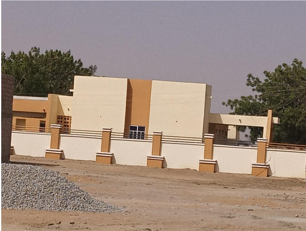
Fig 03: Newly Construction Of staff Quarters in Argungu
