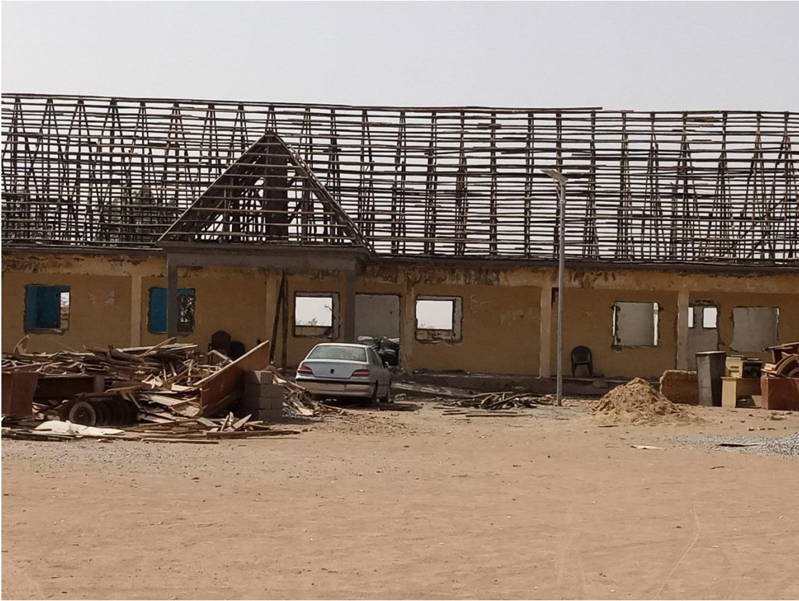
Fig 04: Renovation Of Local Government Secretariat Baudo
