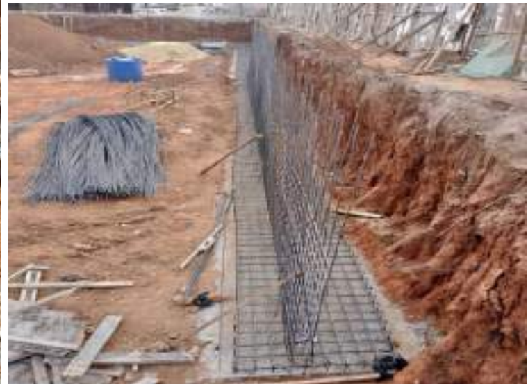
Pic. 4 - Reinforcement of the retaining walls
