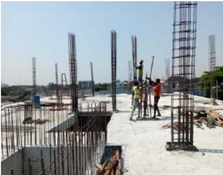
Pic. 7 & 8 – Columns' reinforcement and formwork.
