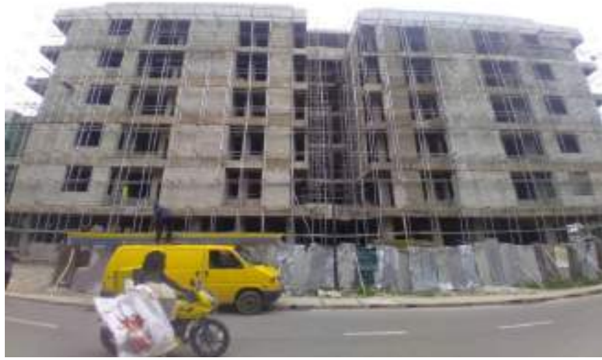
Pic. 11 – Blockwalls ready for rendering
