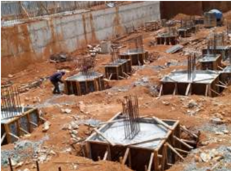
Pic. 3 - Construction of pile caps
