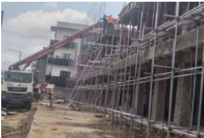
Pic. 9 - Pumping of concrete of the second floor by Lafarge Cement
