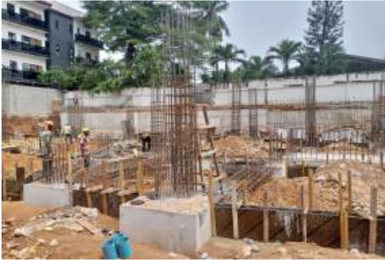
Pic. 5 – Reinforcement of ground beam and column at the basement
