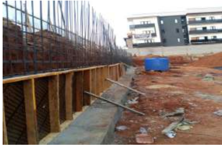
Pic. 6 - Formworks for basement retaining wall
