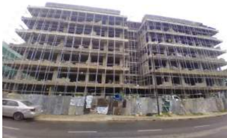
Pic. 10 - Concrete framed structure up to the pent house floor level
