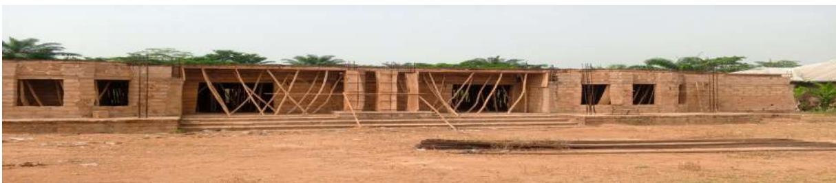
Fig 05: on-going construction Village hall for Umuezeleke ukwakwa Azia
