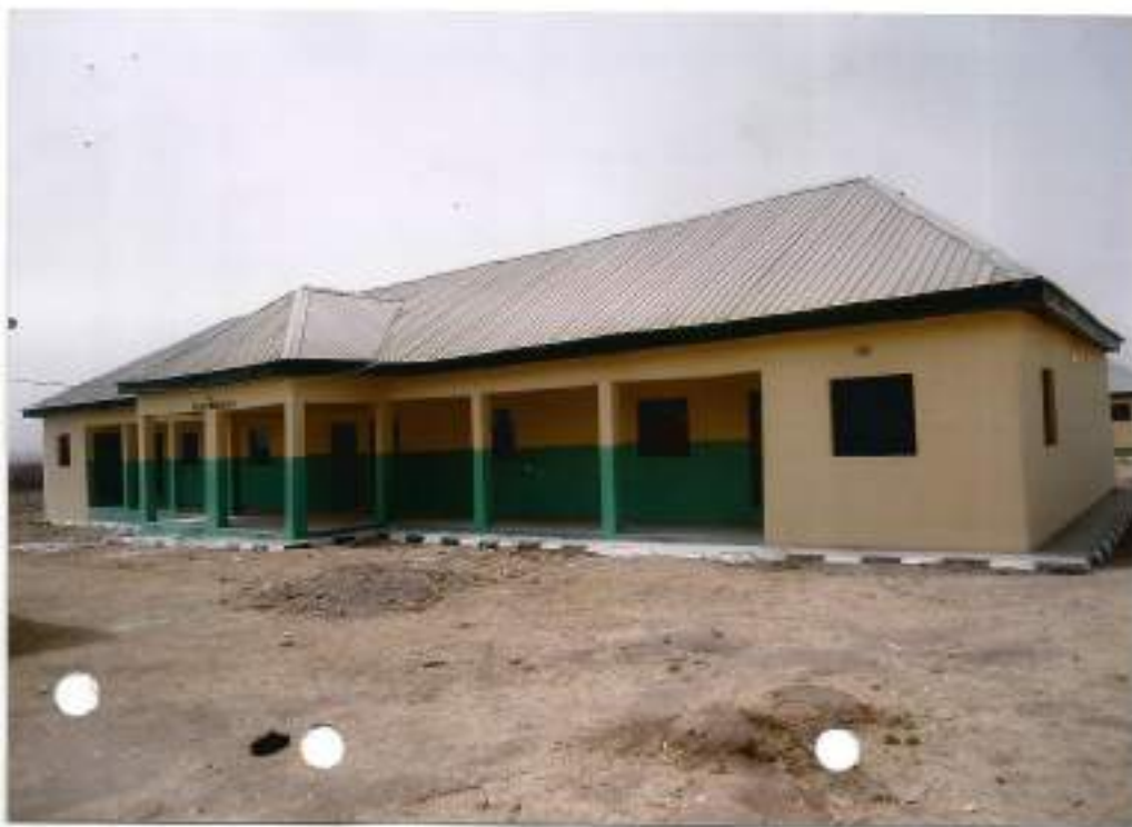
Figure 4. Completed block of Science/Intro Tech Laboratory
