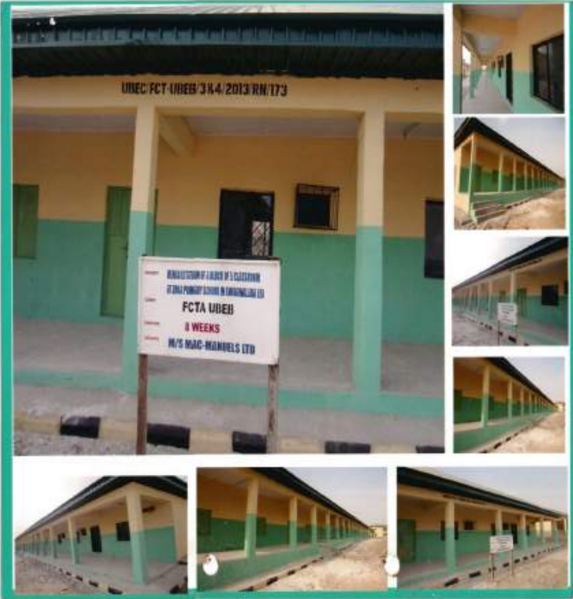
Figure 15. Newly constructed Administrative Block
