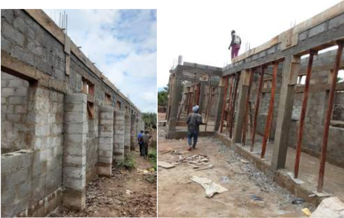
Figure 19. Dilapidated classrooms for renovation
