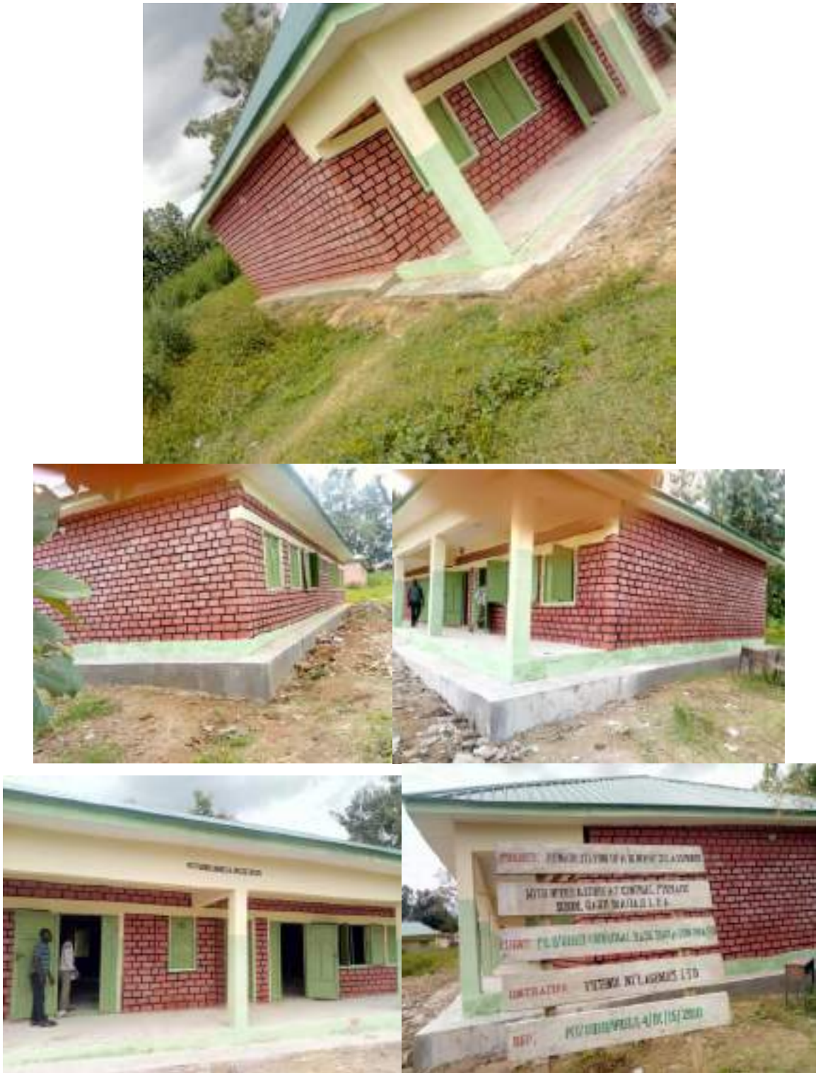
Figure 3. Rehabilitated block of two (2) classrooms with office and store
