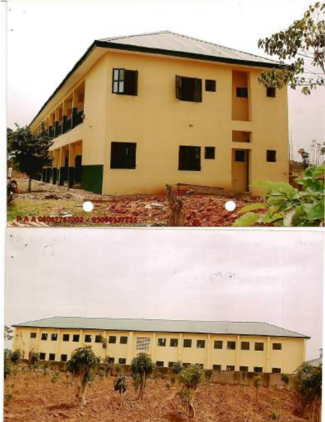
Figure: 7. Construction of a block of three (3) classrooms
