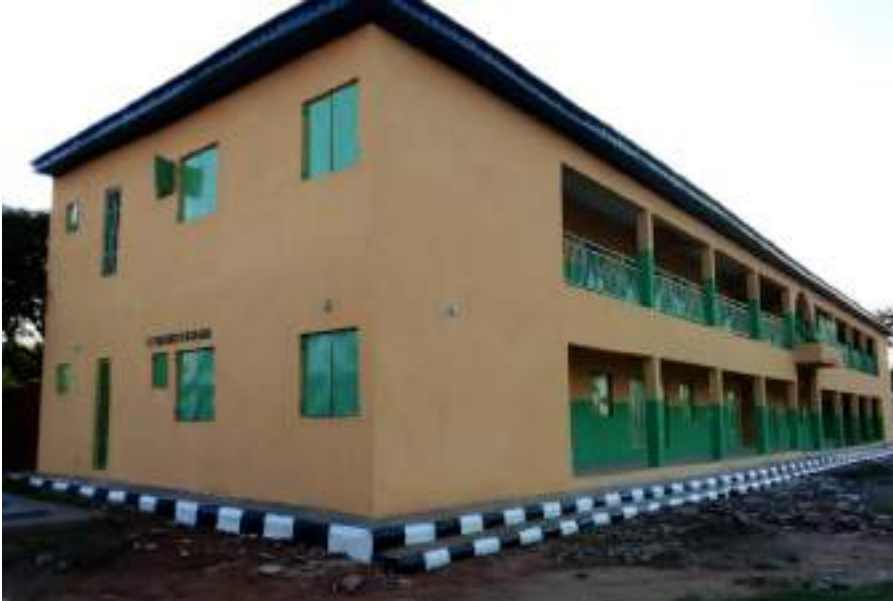
Figure 1. Newly renovated block of eight (8) classrooms
