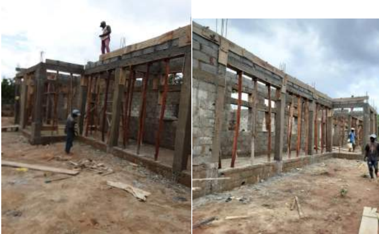
Figure 20. Construction of Science/ Intro Tech Laboratory ongoing
