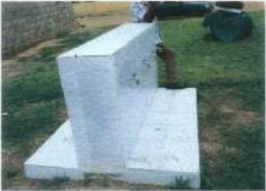
Constructed tap stand in place
