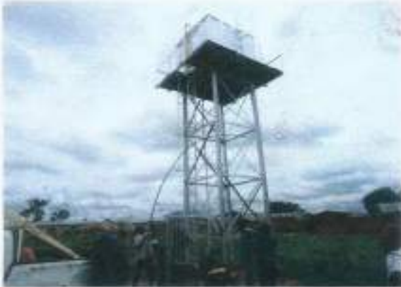
Constructed overhead tank
