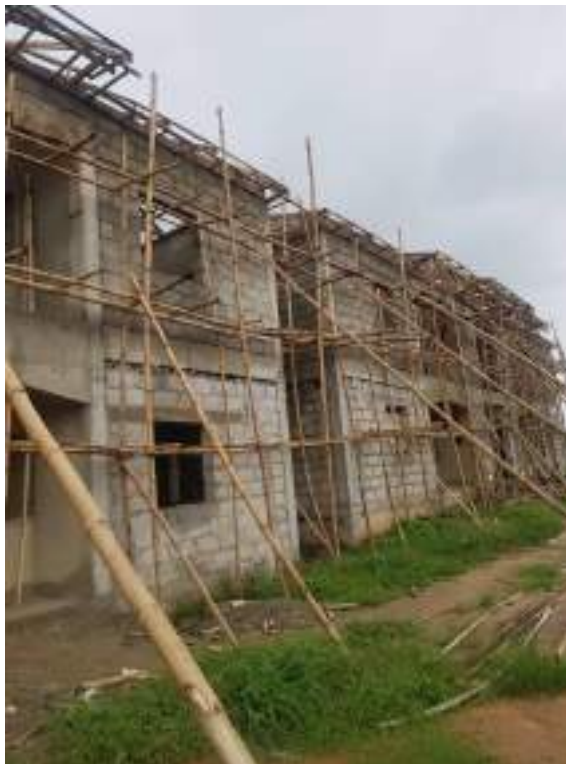
Figure 2. Ongoing construction of eight (8) classrooms (Upstairs)
