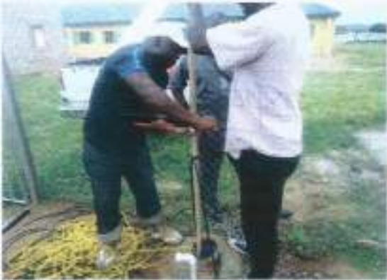
Technicians installing pump
